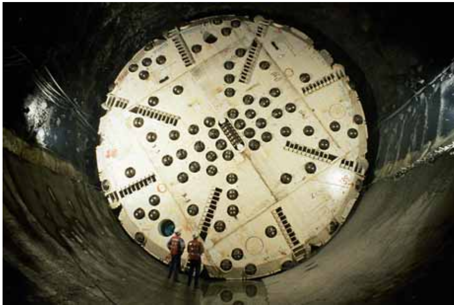
Figure 5 Hsuehshan Main Tunnel TBM Launching
